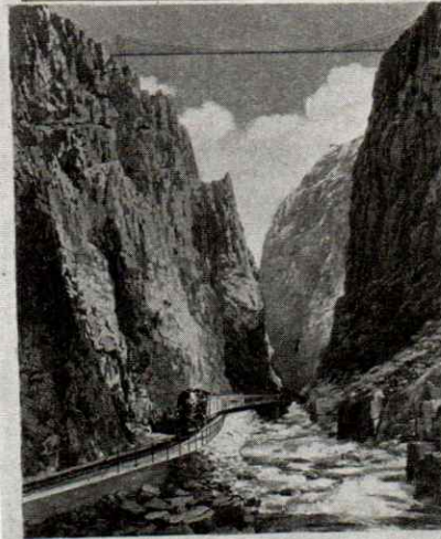
The D. & R. G. "Scenic Limited" in the Royal Gorge—near Canon City
